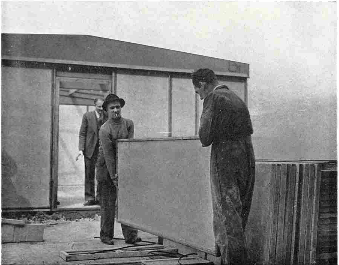
The correct way of carrying a "SECO" Unit from the stack.
