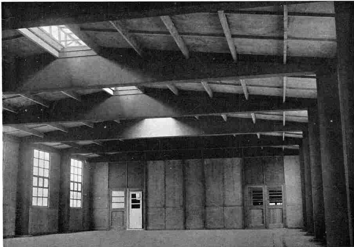
A 35' span high ceiling Workshop fitted with Standard "SECO" Top Lights, one Unit wide extending the whole length of the 12' bays.
