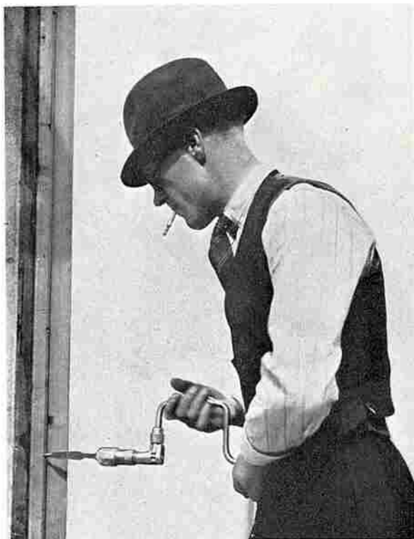
Screwing a Door Frame to the adjoining Unit.
