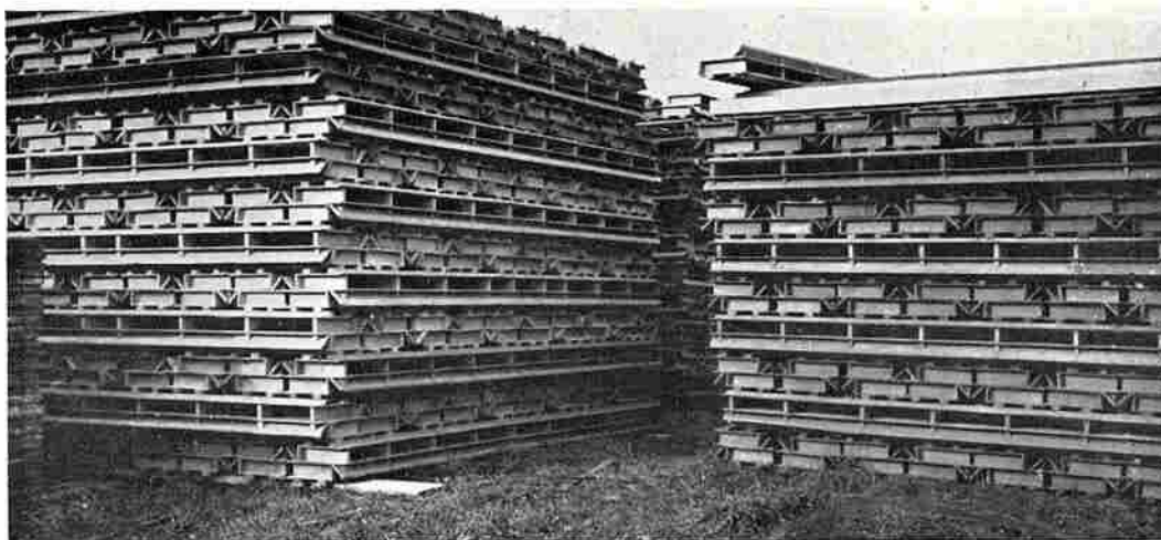
A neat pile of Type "A" Eavespieces — weather mouldings carefully protected by alternate stacking. Cover with Tarpaulins to protect from wet and sun.
