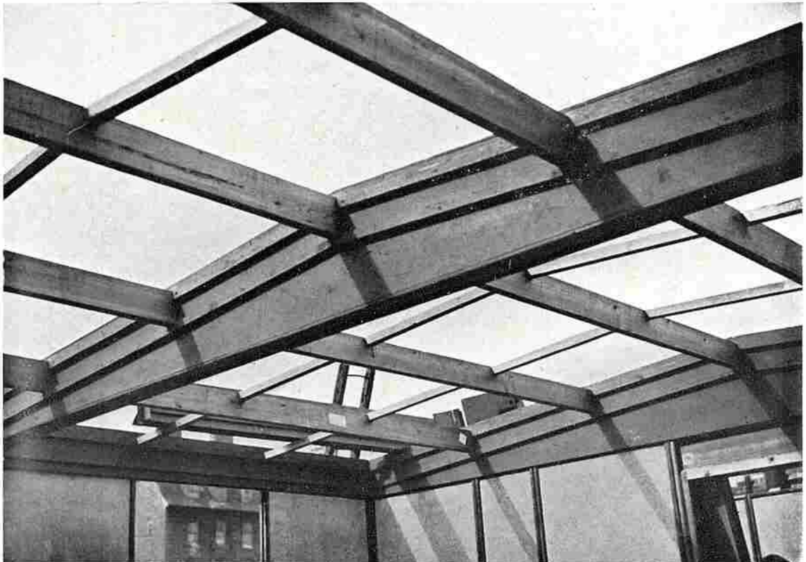
The roof structure ready to receive the Roof Units. Roof Spars are in position in the slots on beam faces and roof ties act as cross bracing.
