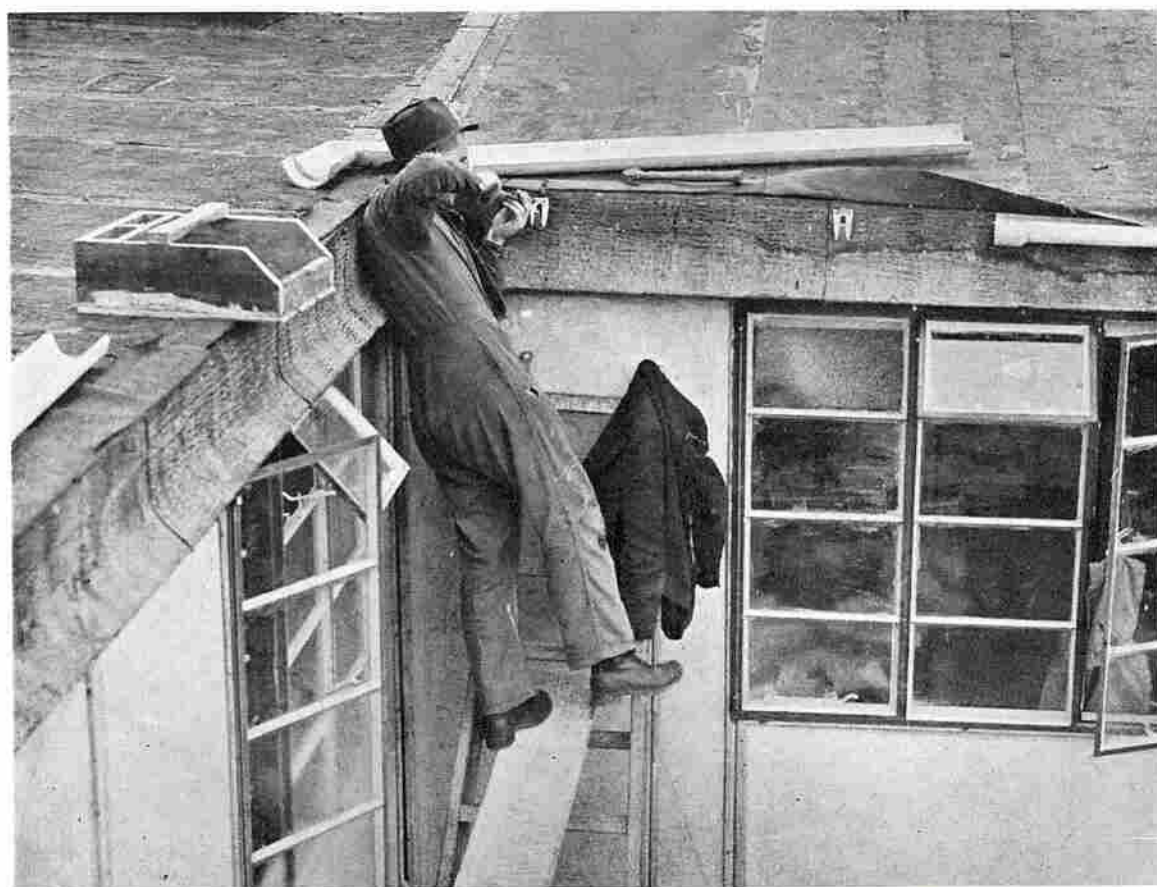
If guttering is required, it should be fixed above the Weather Mould of Eavespieces, and the top layer of felt dressed into the gutter.
