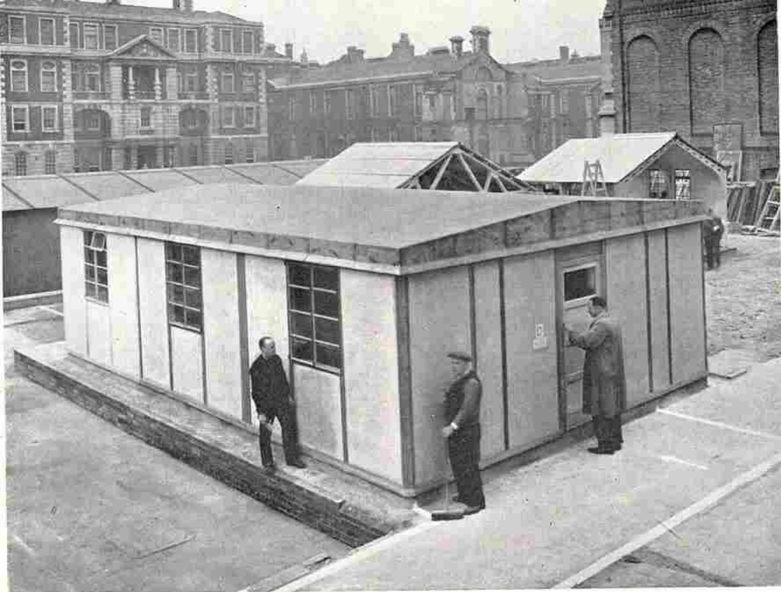
The building is complete, with the Roofing Felt applied. Note the clean finish of the Felt at Eaves and Weather Drip.
