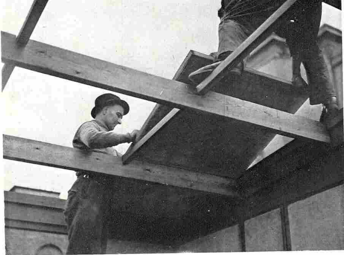
A Roof Unit being lowered into position. WARNING.—The Operator is disobeying instructions by standing on the 2" x 2" Roof Tie. He is risking a serious accident.
