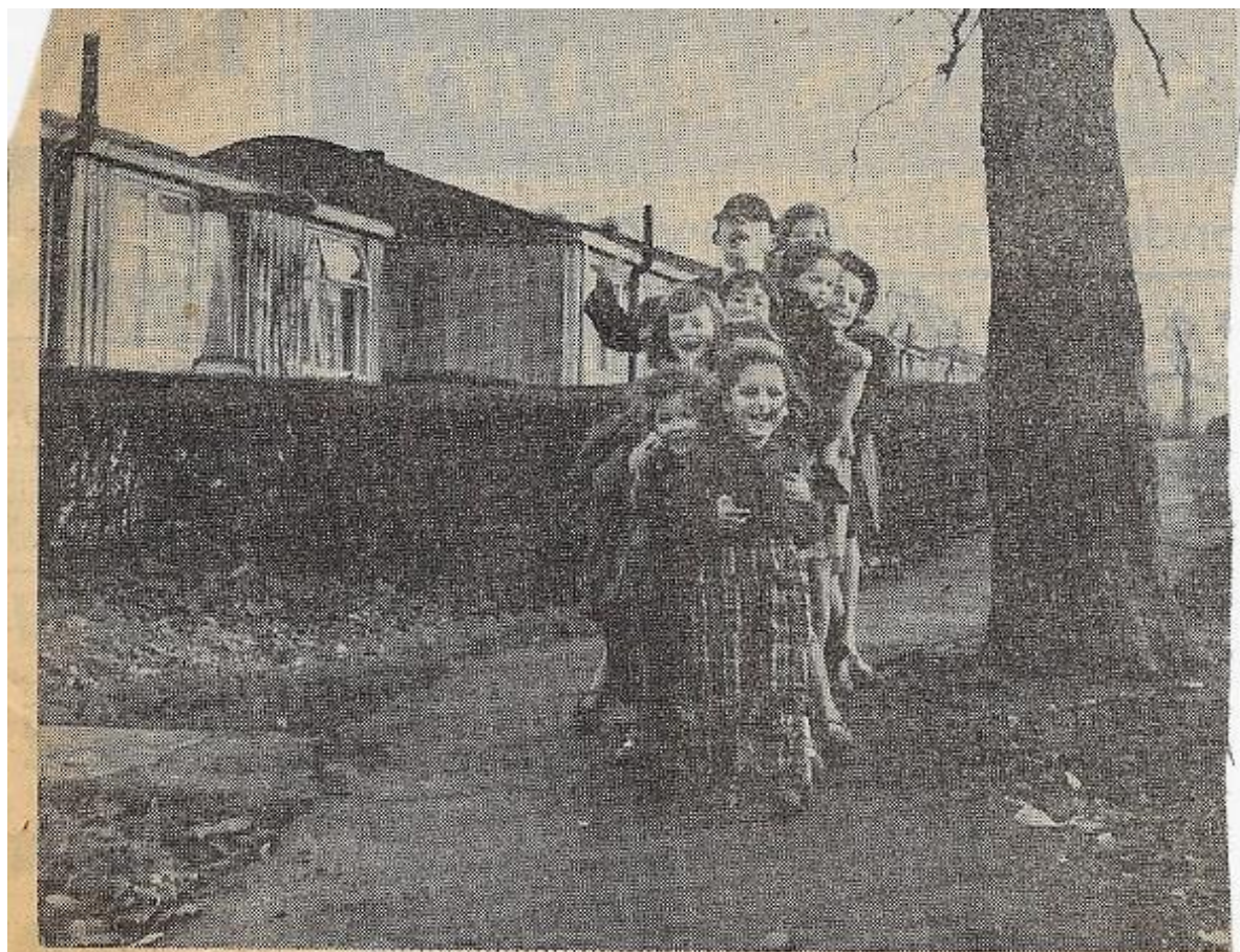
To the adults the prefabs have been a temporary expedient to help solve the post-war housing problems, but to the children shown here, outside the Kingsbury-road row which is next on the Council's programme for demolition, the little bungalows have always been "home."
