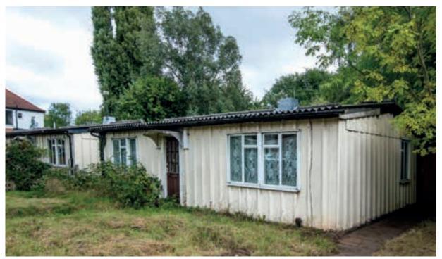
The Phoenix prefab was designed by Laing with its partners McAlpine and Henry Boot. It has a steel frame and is clad with corrugated asbestos cement sheets with a tubular steel roof. Each Phoenix prefab cost £1200 to produce. A specially insulated version was manufactured for the Isle of Lewis in the Outer Hebrides at a cost of £2000 each.
