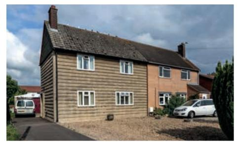
The Burt Committee produced a number of reports on permanent prefabs, which were described as Official Permanent Prefab Houses. The permanent prefabs were two storey houses with steel or concrete frames clad with precast reinforced concrete (PRC) panels, with the exception of the Hawksley BL8 bungalow.
