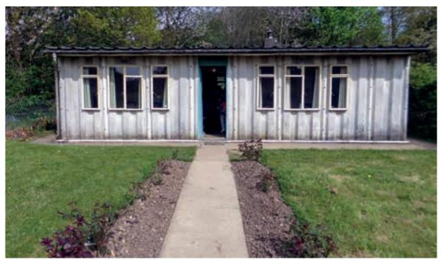
The Universal prefab was manufactured by the Universal Housing Company of Rickmansworth in Hertfordshire. The Universal Housing Company had constructed many non-traditional houses using prefabricated sections before the Second World War.
