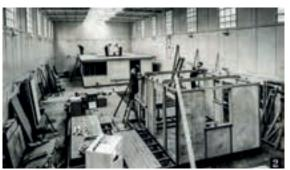
Prefabrication is a method of producing standardised components off-site in a factory, that can be fitted together on-site. The components can be shipped flat packed or partially assembled and are not subject to weather conditions when they are manufactured.
